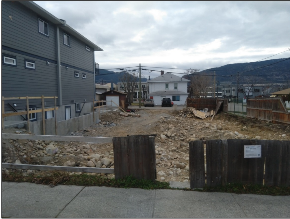
Figure 4: East View (from Van Horne Street)
